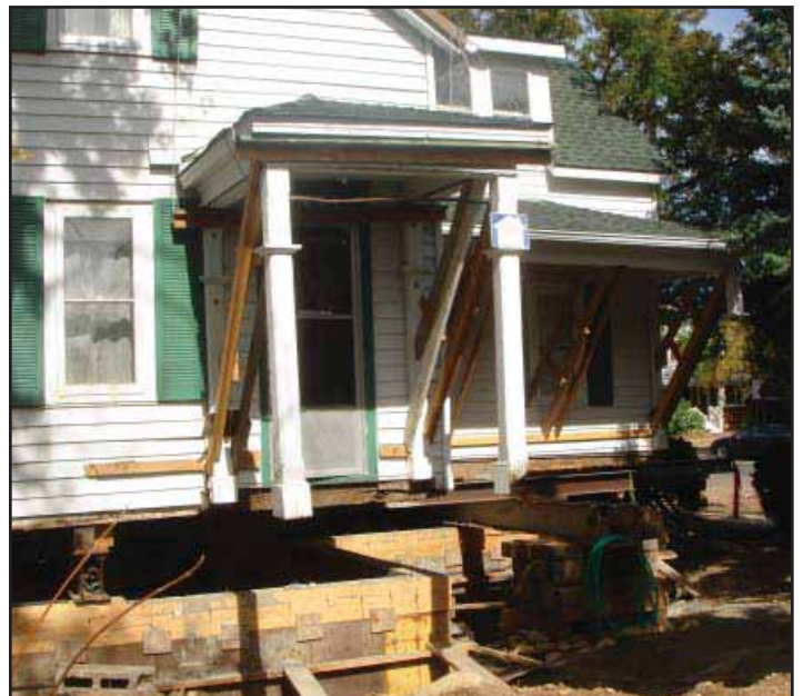
Site the structure in the same direction as exemplified by its original location. This building has been relocated, but both the front entrance and side doors are oriented toward the street as before. Boulder, CO
