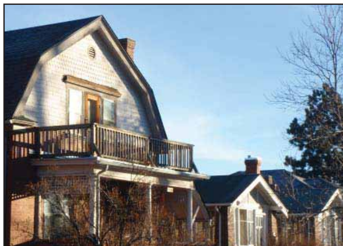
The new roof on this building is not in keeping with the scale and massing of other buildings on the same block and overwhelms the original structure. Denver, CO
