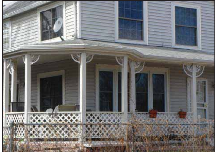
The architectural detailing of this porch is overly ornate and not in keeping with the architectural style of the house. Denver, CO
