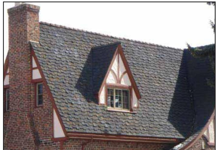
*The thickness and uneven dimensions of this asphalt shingle roof mimic traditional wooden shingles. Denver, CO*
