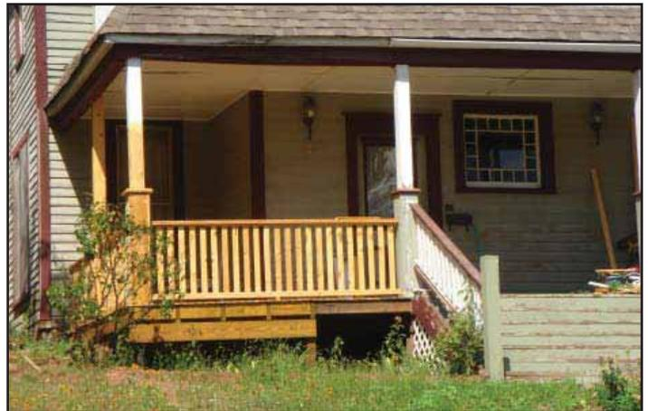
*The porch reconstruction project includes posts, railings and pickets that are similar in form and material to the original, missing pieces. Manitou Springs, CO*
