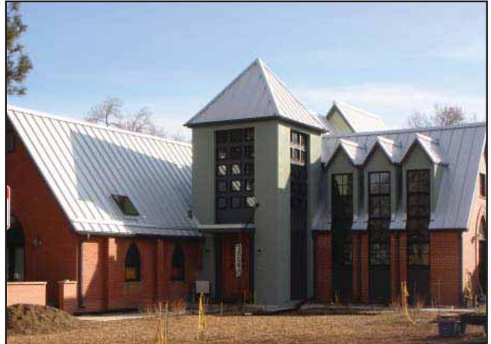
*This standing-seam metal roof contrasts with the historic architectural style, is highly reflective and is generally not permitted. Denver, CO*
