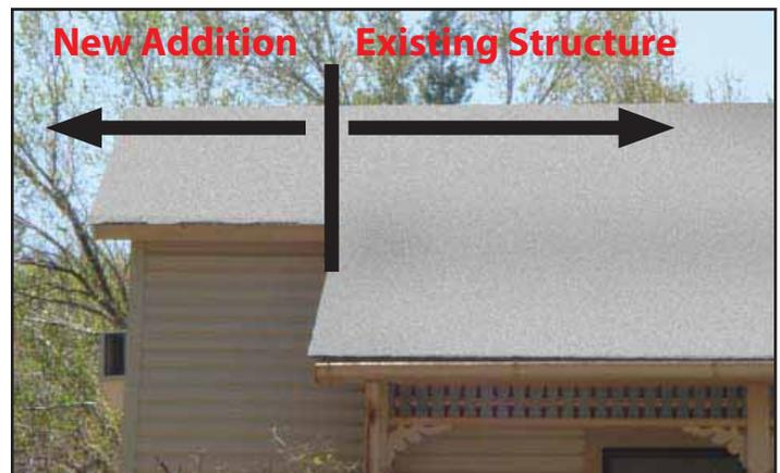
*The addition to this house used similar materials to minimize the visual impact of the addition to the original structure. Manitou Avenue, Manitou Springs, CO*
