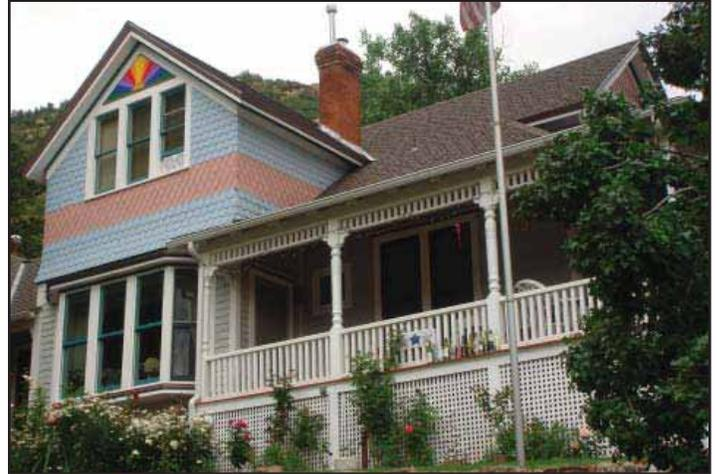
*The building materials on this house include shingles, clapboard, wooden trim and lattice. When undertaking an addition or alteration, it is important to maintain a similar materials palette and match the proportions of each material as seen on the original structure. Manitou Springs, CO*
