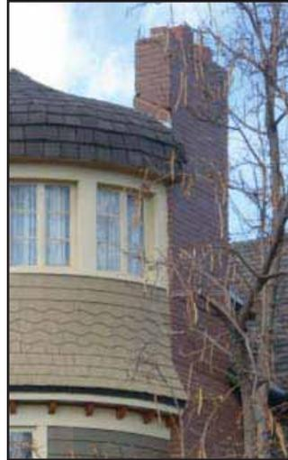
The chimney on the left has been covered with siding during a recent alteration project and conceals the original brick, which provided visual interest from the street. The chimney on the right has been tuck-pointed during recent renovations. Denver, CO
