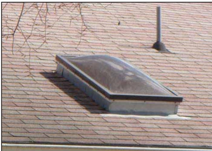
Avoid locating skylights on roofs visible from street; this is a photograph of a "bubble skylight", which is not permitted.
