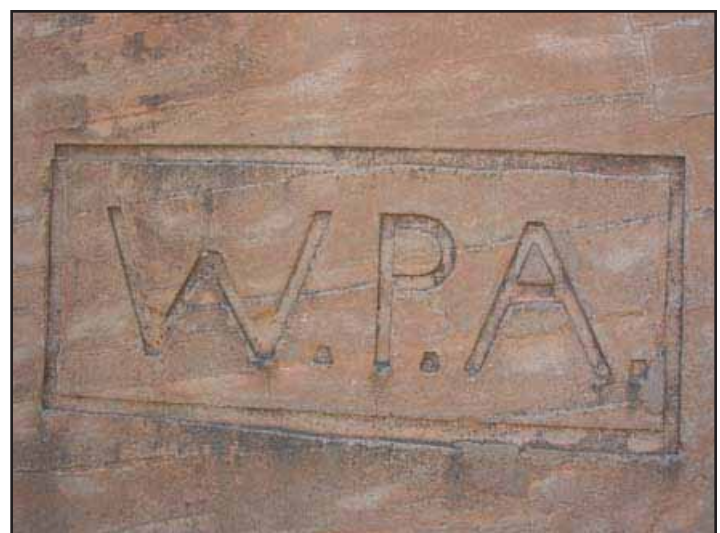
The WPA insignia on a retaining wall in the Upper Washington Subdistrict. Lafayette Avenue, Manitou Springs, CO
