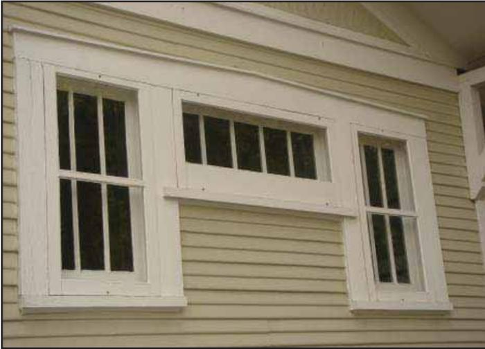
*The City of Manitou Springs advocates the maintenance and repair of windows on contributing structures. This original window includes exterior storm windows that are removed in the warmer months. Denver, CO*
