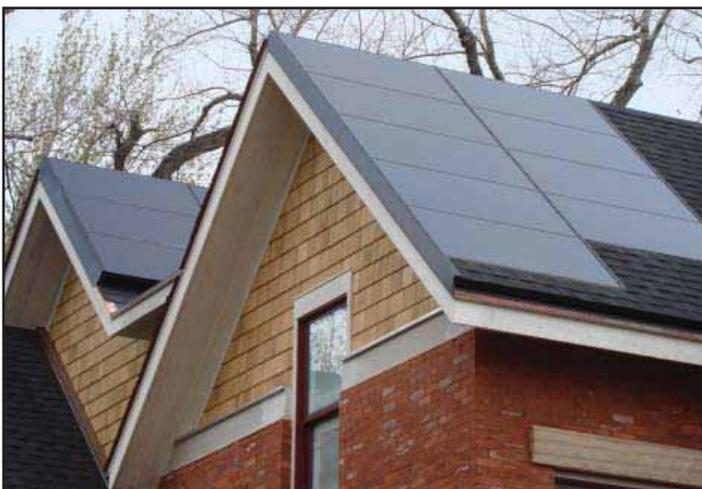
*This new residence in Boulder includes photo-voltaic cells mounted at the same angle as the roof to match the profile of the roof. Boulder, CO*
